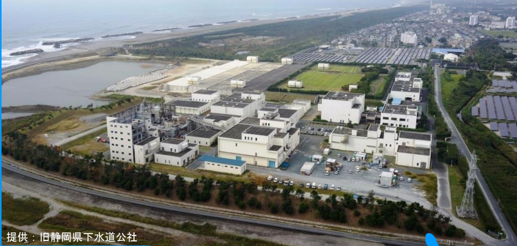
SEIEN Sewage Treatment Plant
